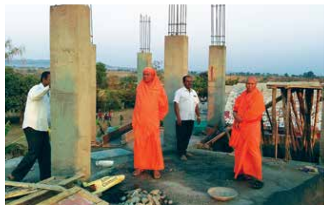
Our coordinators inspect the progress of construction.
